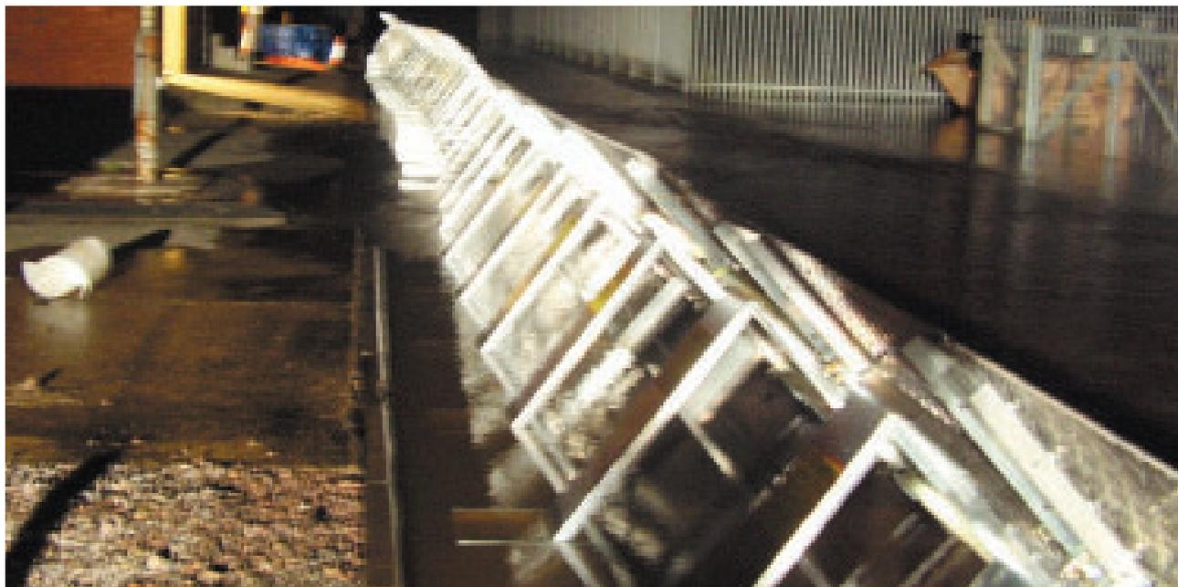
Temporary defences set up to protect Walham electricity switching station – preventing around 450,000 domestic and commercial customers losing power
