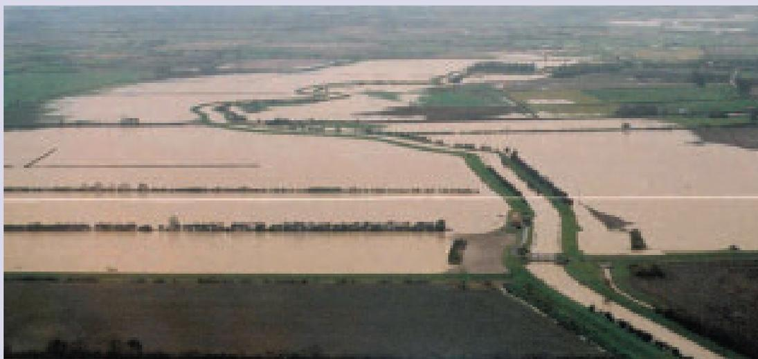
Till washland in flood – the embankment and control sluice (foreground) hold back the water from passing downstream to Lincoln.
