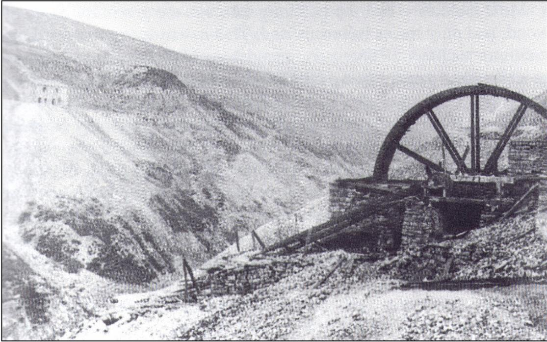
Plate 2.3: Water-powered crusher, Bunton Level, Gunnerside Gill (from Morrison, 1998)
