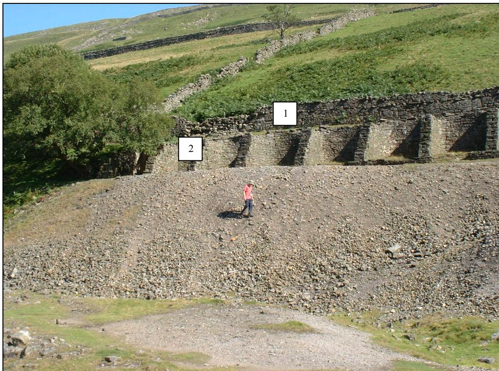
*Plate 2.2: Bouse teams, Old Gang Company dressing floor, Sir Francis Level, Gunnerside Beck. Water was channelled behind the structures (1) and through each individual bouse team (2)*
